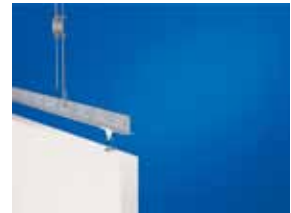
Solo Baffle/hook installation
